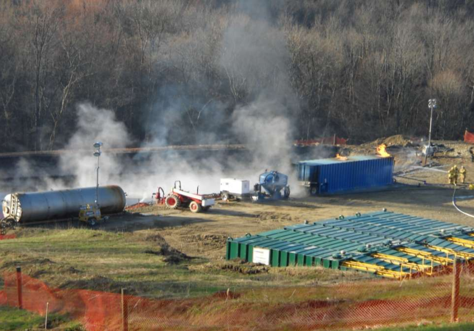
Fracking Pond Fire – Hopewell Township, PA – April 1, 2010
